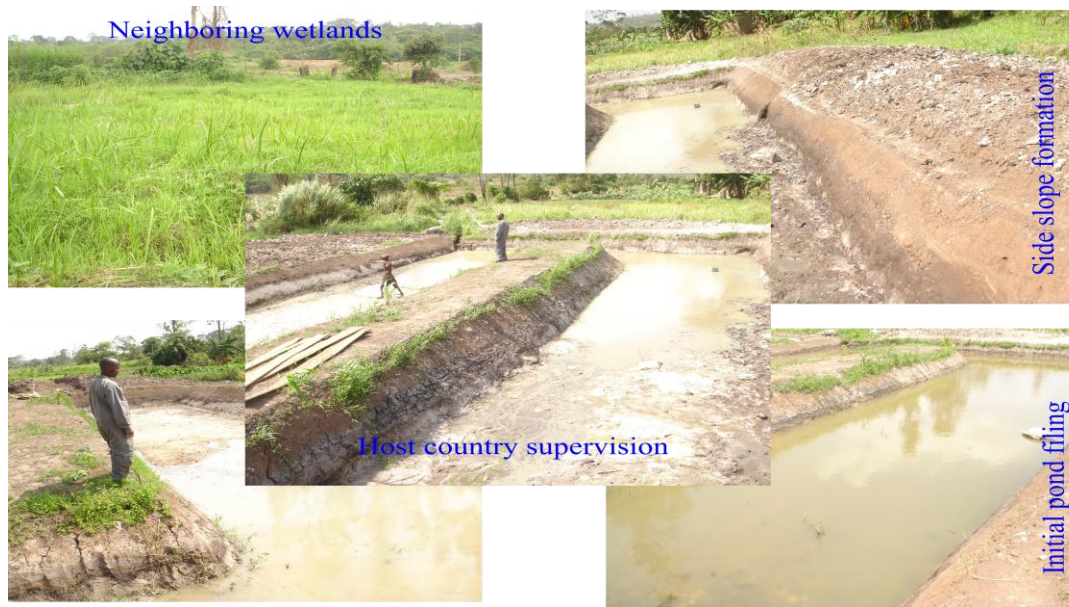
Figure 3: Photos of pond construction site, neighboring wetlands, and agricultural activities
