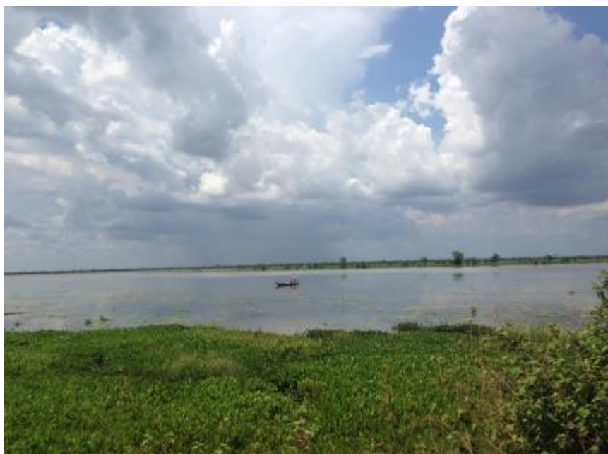
Figure 1. Stung Chinit Reservoir in Kampong Thom province.
