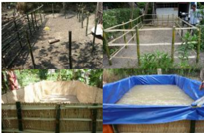
Designing plastic lined-tank
