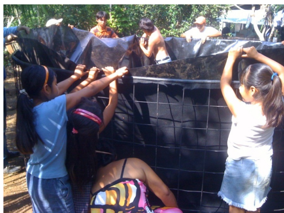
Assembling geomembrane tank for fish
