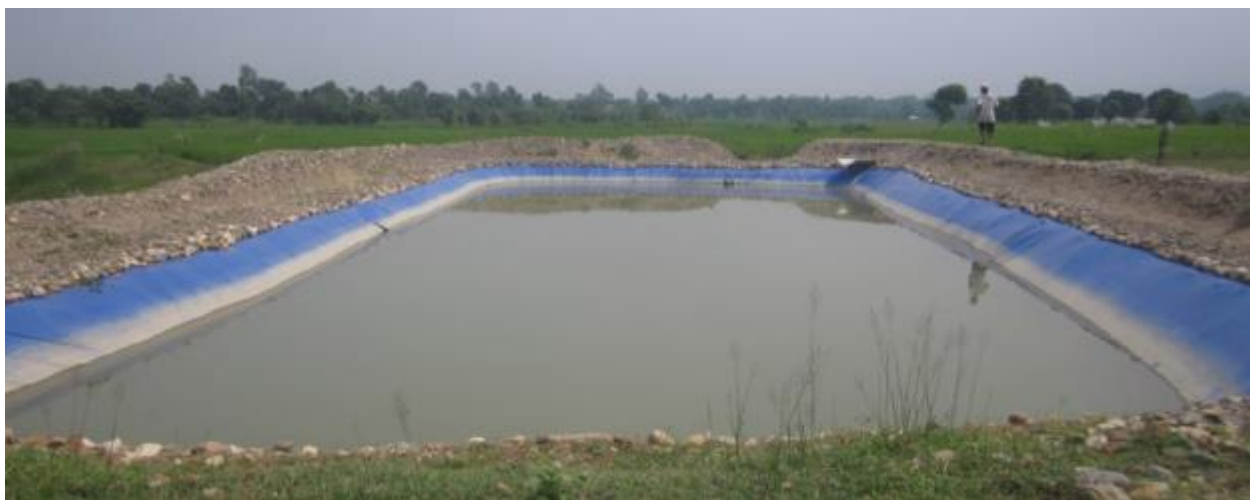
Figure 4. Fish pond constructed at Janta Higher Secondary School, Kawasoti.
