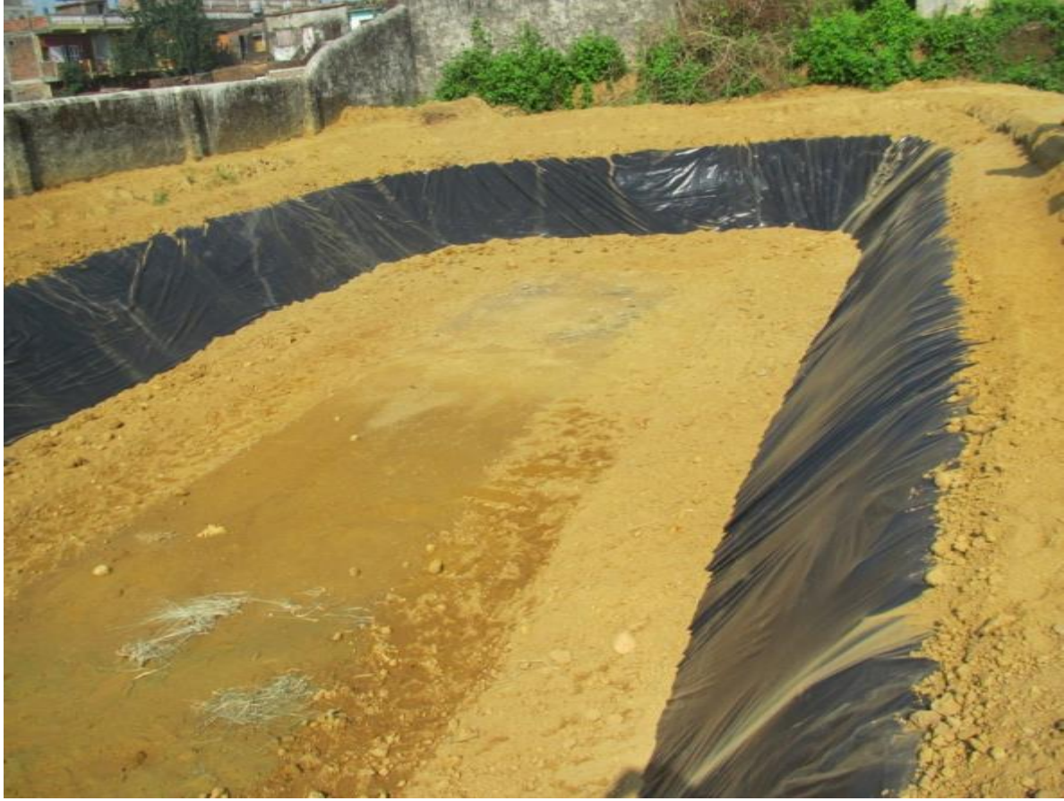
Figure 2. Fish pond constructed at Nepal Higher Secondary School, Tandi.
