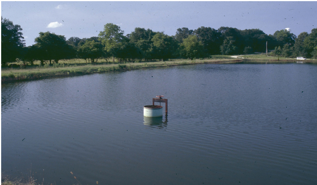
Figure 1. Photograph illustrating the drop-fill method for water replacement. When water is added to restore evaporation and seepage losses, the water level is not increased to the level of the overflow intake to provide capacity to store rainfall and runoff.
