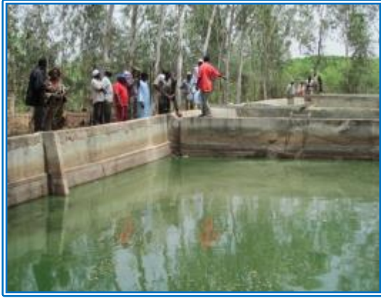
Tanks originally constructed for other purposes can be used for fish production, as practiced by farmer Mafa Fofana.
