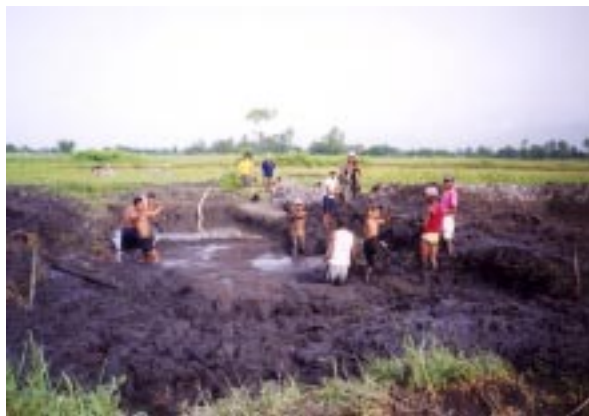
New earthen ponds under construction at IAAS.
